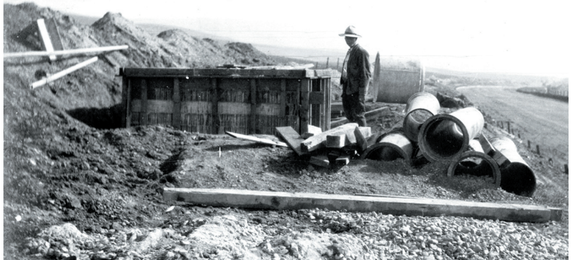
Construction of District's water distribution system, circa 1926
